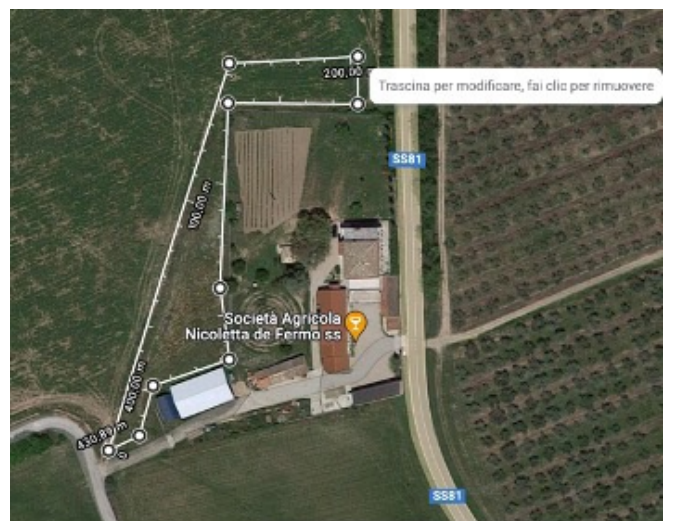
Aerial photo with site localization - tot area: 3035 sqm
